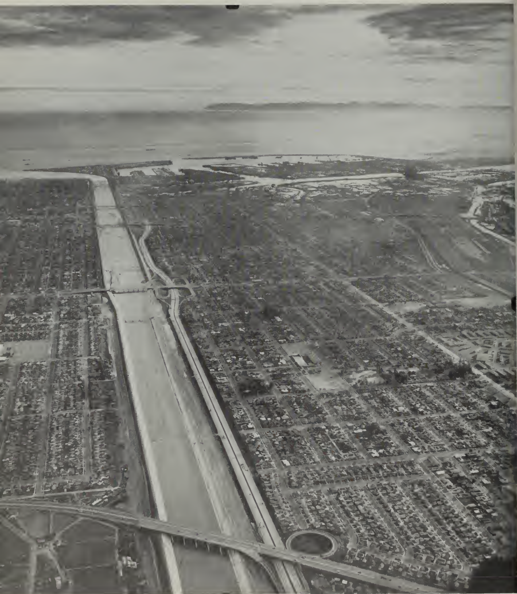
South Coastal Area—Los Angeles River
